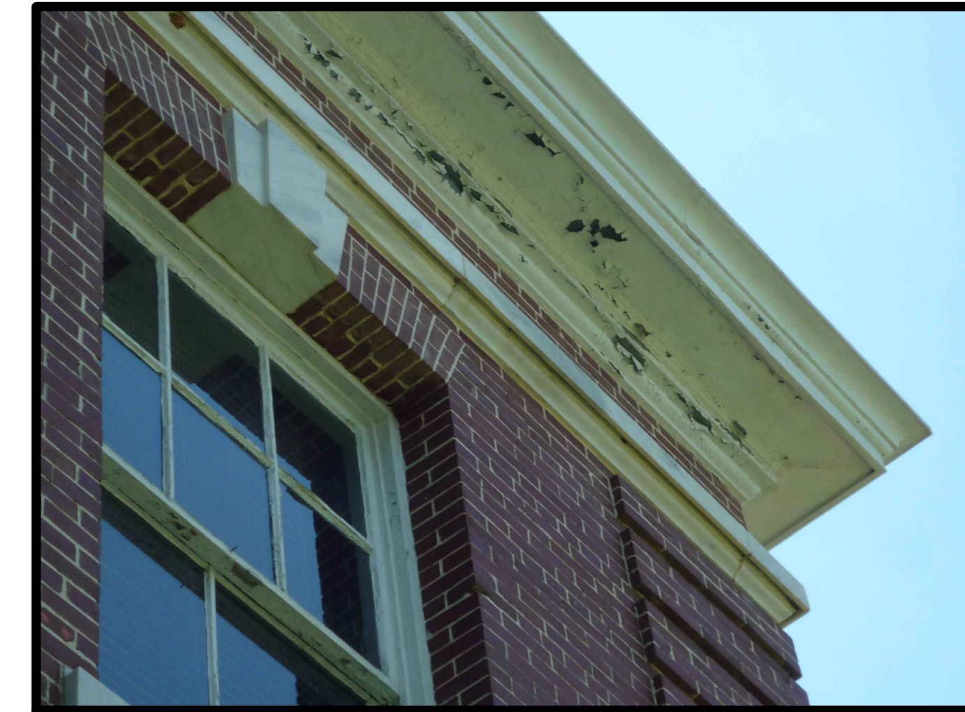
TYPICAL PAINTED METAL AT ROOF EAVE
