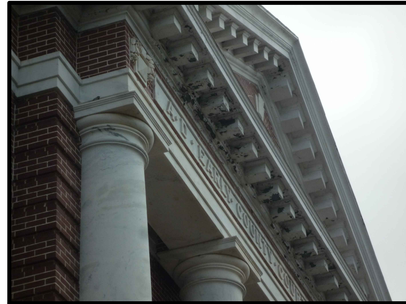
TYPICAL PAINTED METAL AT ROOF GABLE
