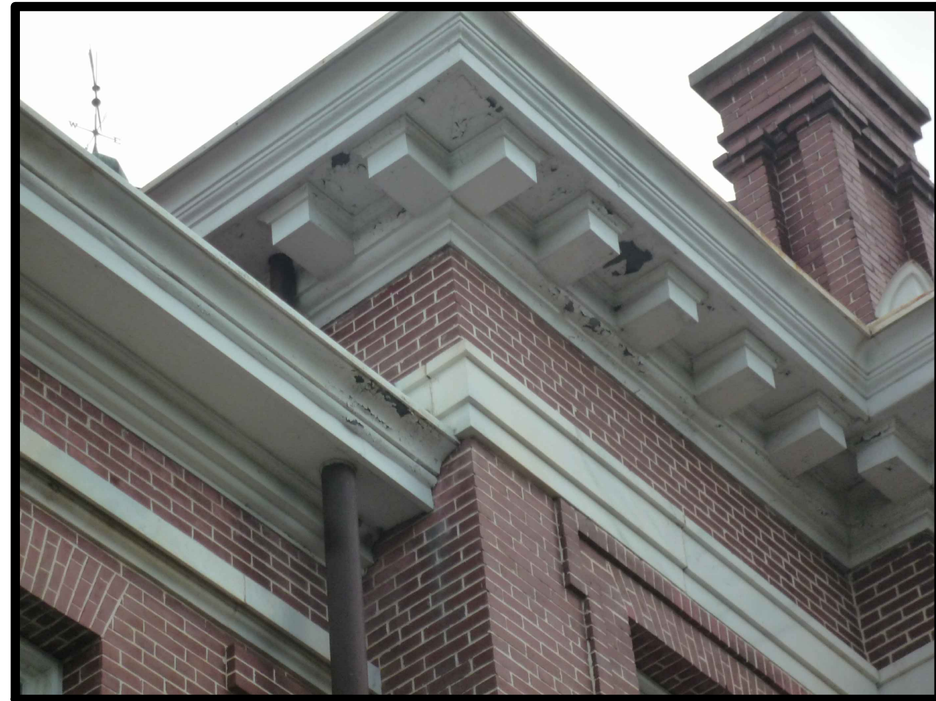
TYPICAL PAINTED METAL AT ROOF EAVE
